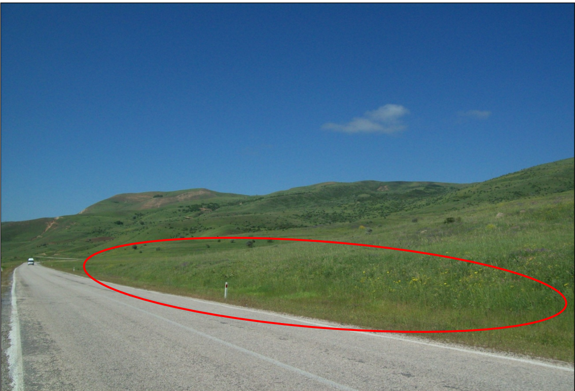
Figure II.8. General View of the Storage Areas (D1, D2 and D4)
